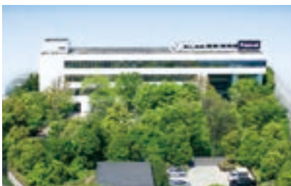
Head office / R & D center
